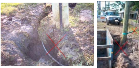
Above: Poles with become unstable if undermined
